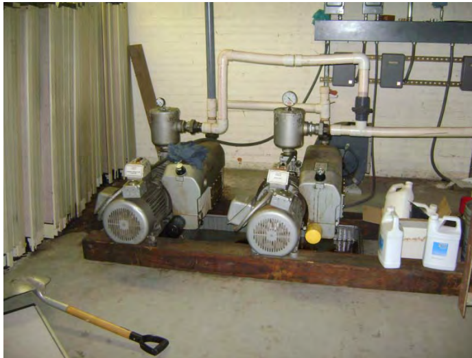
Photograph 7: Basement vacuum pumps and drip pans
