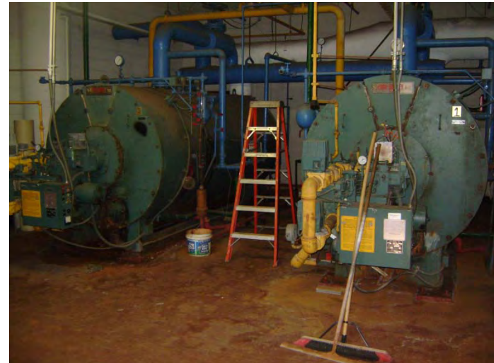
Photograph 4: Basement boiler room with two gas-fired boilers
