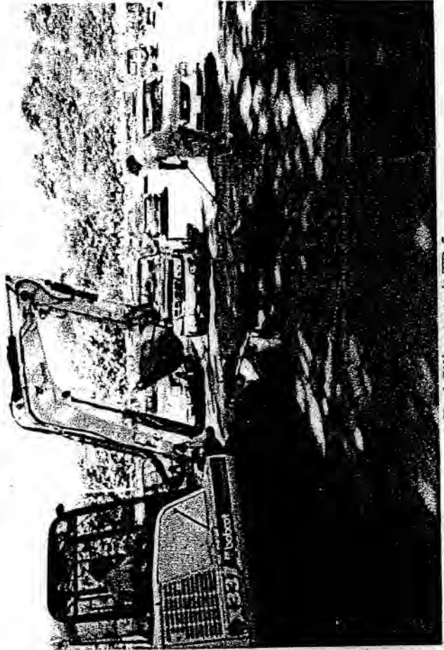
Backfilling test pit TP-5
