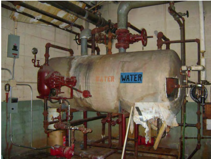
Photograph 9: Basement condensate room and tank
