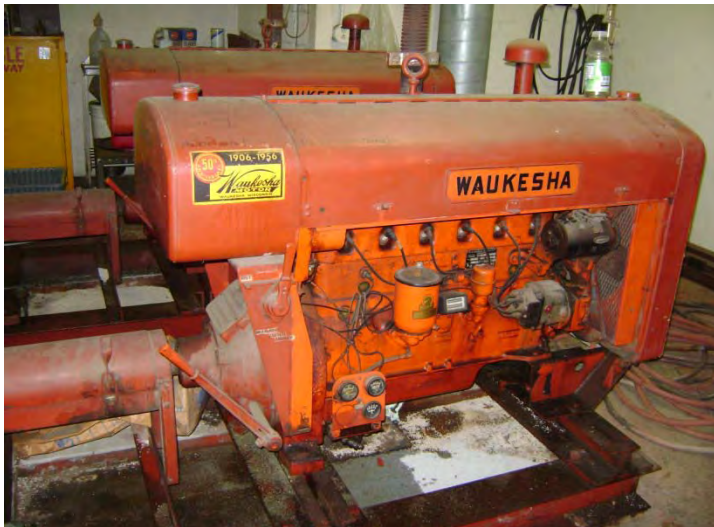
Photograph 11: First floor flood control pump engine – original equipment.
