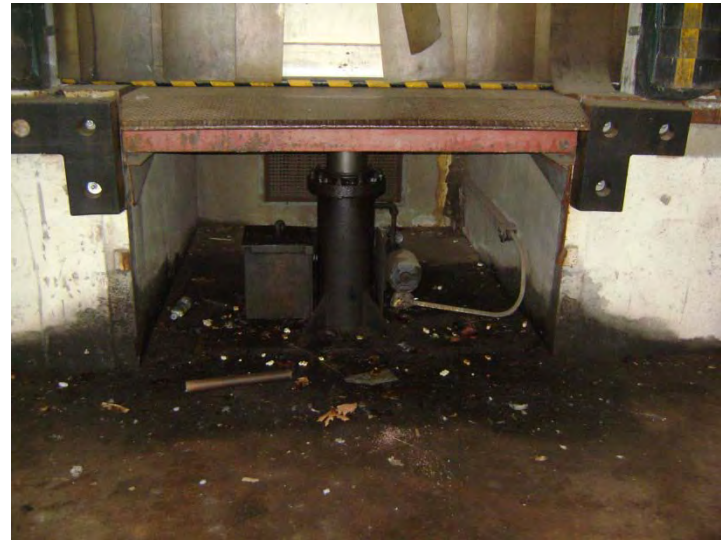
Photograph 14: Loading dock leveler
