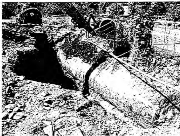
Excavating the UST
