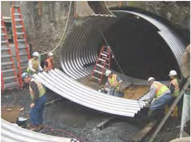
Drainage Culvert, Naugatuck (Source: ADA, Bridgeport CT)
