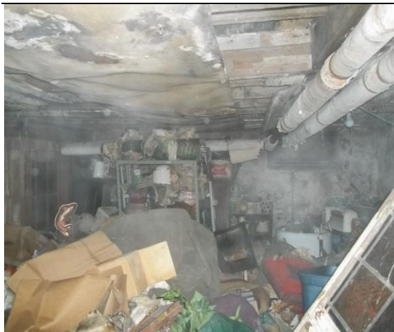
Photo #7: Aircell insulation and stored materials in basement
