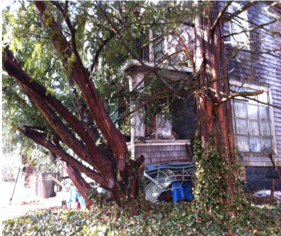
Photo #1: Front of building
