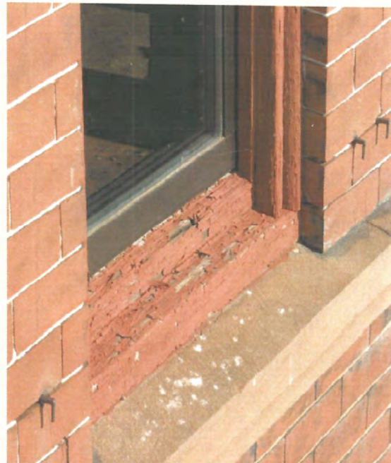
Poor Condition of Wood Conditions
