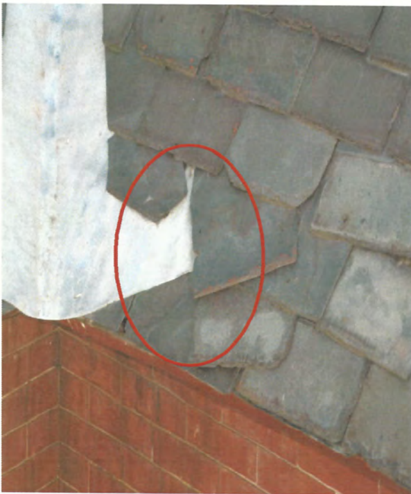
Loose or Missing Slate
