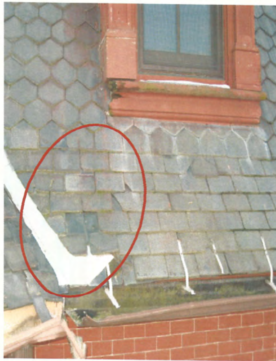
Loose or Missing Slate
