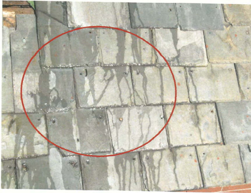
Repairs with used Slates
