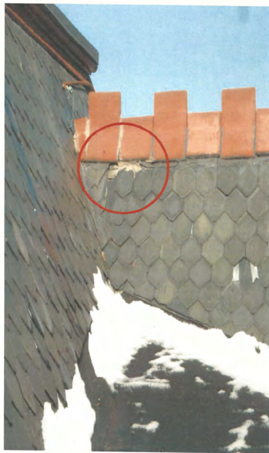
Exposed Wood Plank Deck
