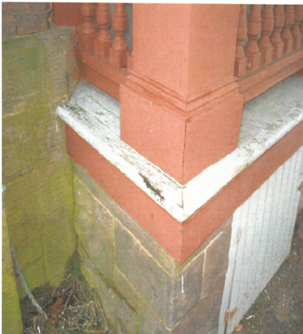
Poor Condition of Wood Conditions
