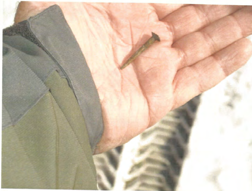
Nails do not meet Industry Standards
