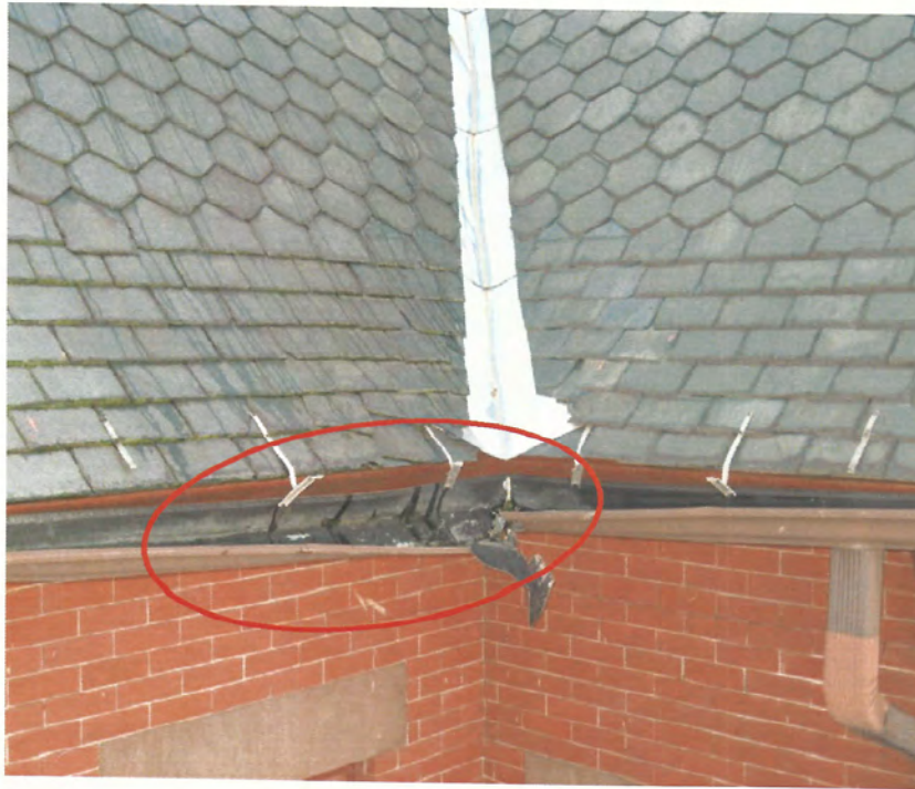
Damaged Gutters
