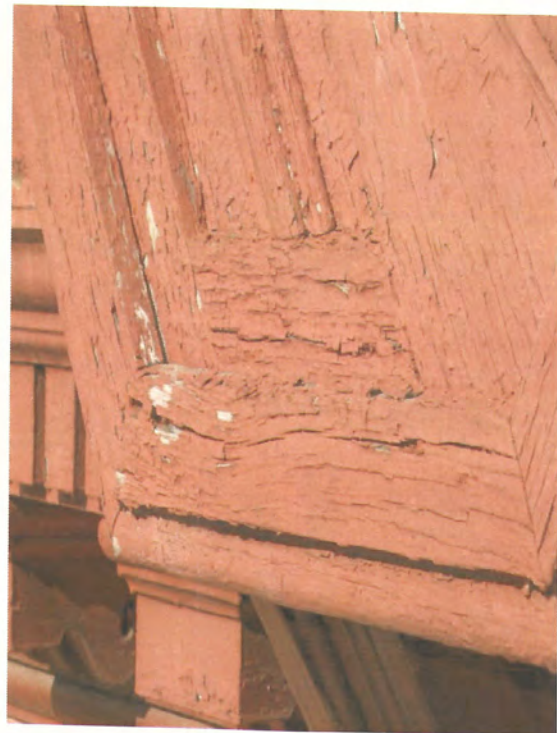
Dried Wood and Peeling Paint
