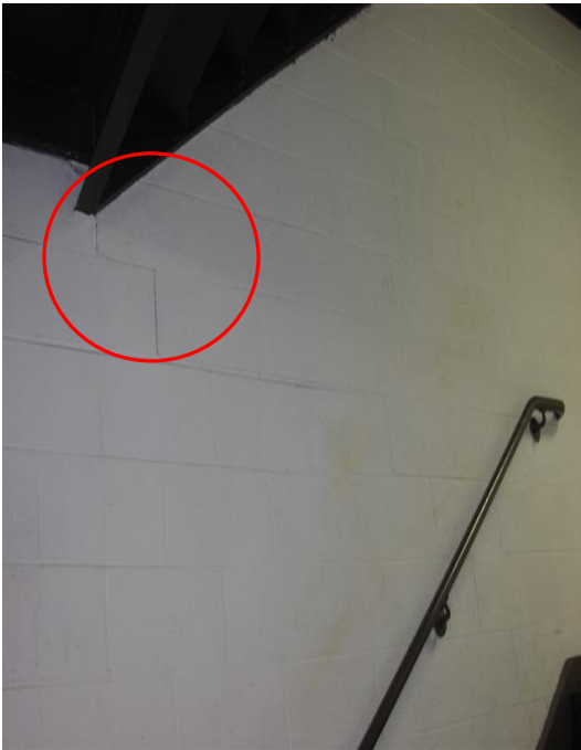
Cracks and Movement in the East Goodyear House Stairwell
