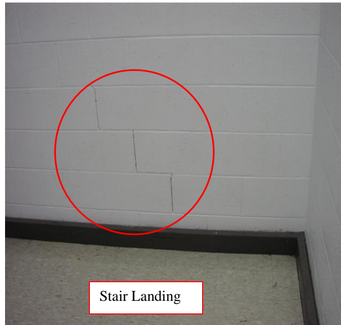
Cracks and Movement in the East Goodyear House Stairwell
