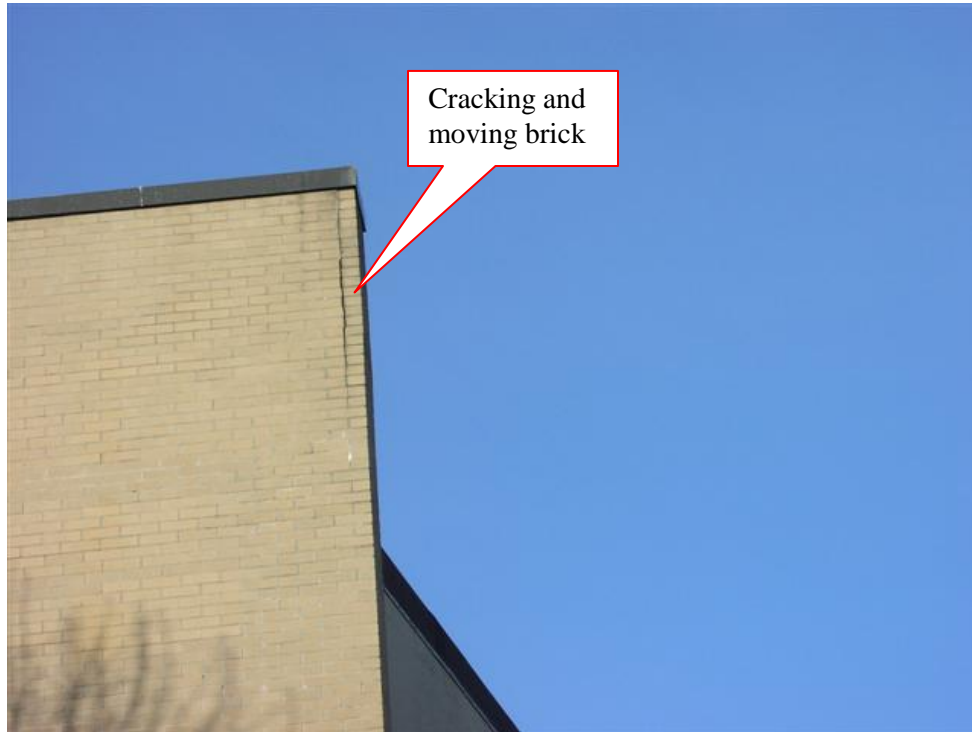
Condition of Exterior Masonry at Southeast corner of Auditorium
