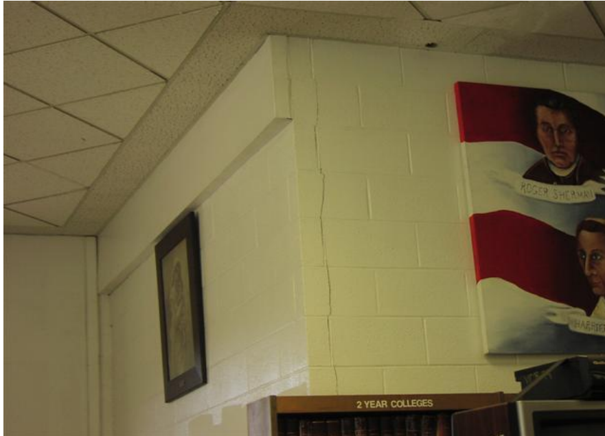
Crack in Media Center Wall
