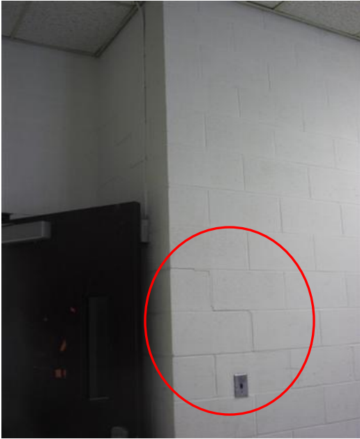
Cracks and Movement in the East Goodyear House Stairwell
