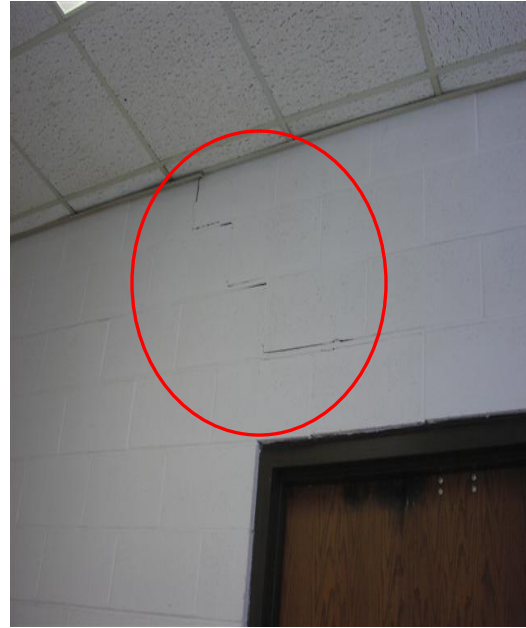
Cracks and Movement in the East Goodyear House Stairwell
