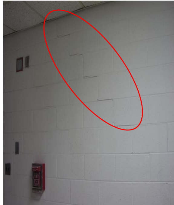
Cracks and Movement in the East Goodyear House Stairwell
