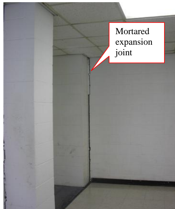
Mortared Expansion Joint in East Connector
