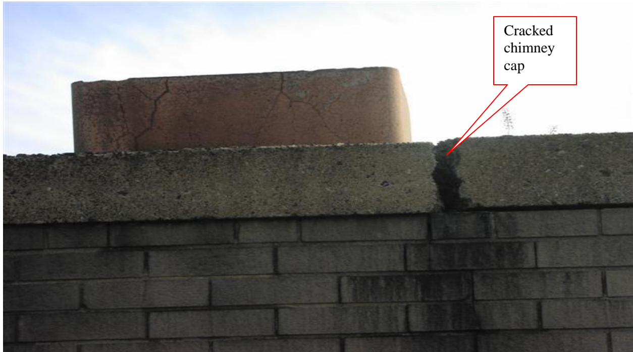
Close Up of Cracks and Movement in West Face of Chimney
