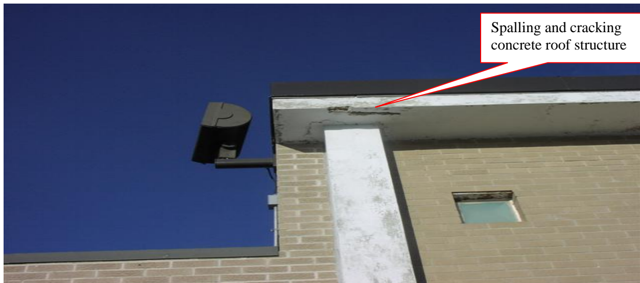
Close up of Spalling Condition
