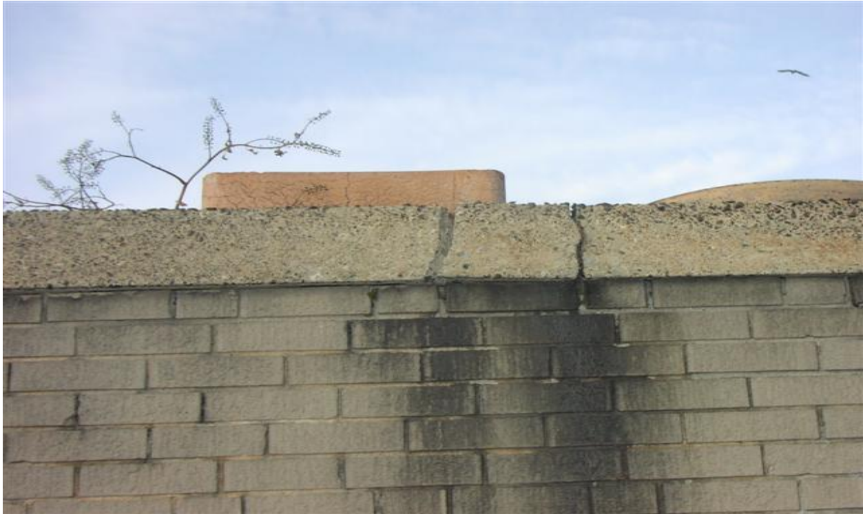
Close Up of Cracks and Movement in East Face of Chimney
