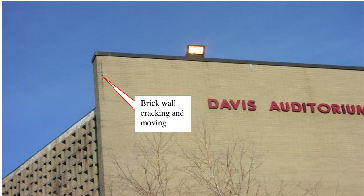
Condition of Exterior Masonry on South Wall of Auditorium
