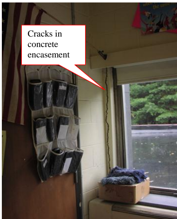
Interior Conditions at Column Encasement
