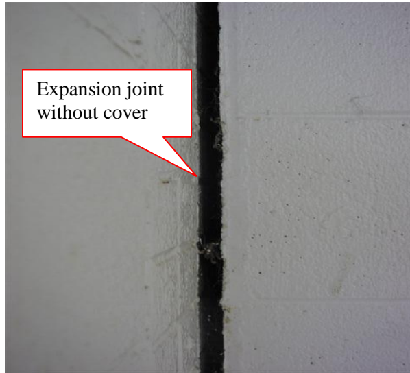
Close up of Joint at Column Enclosure in Upper Level of East Connector
