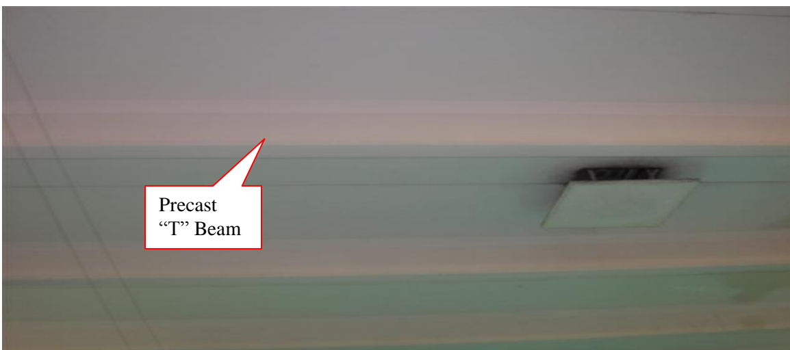
Natatorium Roof Framing
