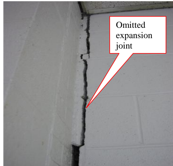
Close up of Mortared Joint at North Wall of East Connector
