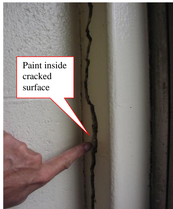
Interior Conditions at Column Encasement
