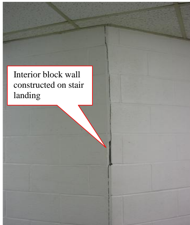
Cracks and Movement at West Stair in Original Building
