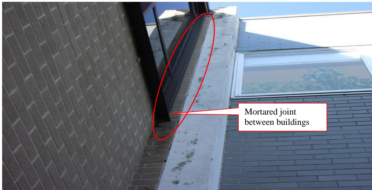
Mortared Expansion Joint between West Connector and Original Building
